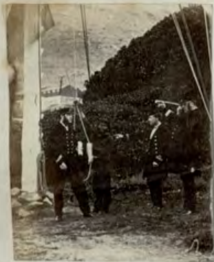
"Hoisting the appurtenances"
