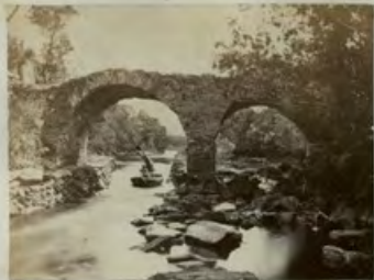
THE OLD WEIR BRIDGE, KILLARNEY.
