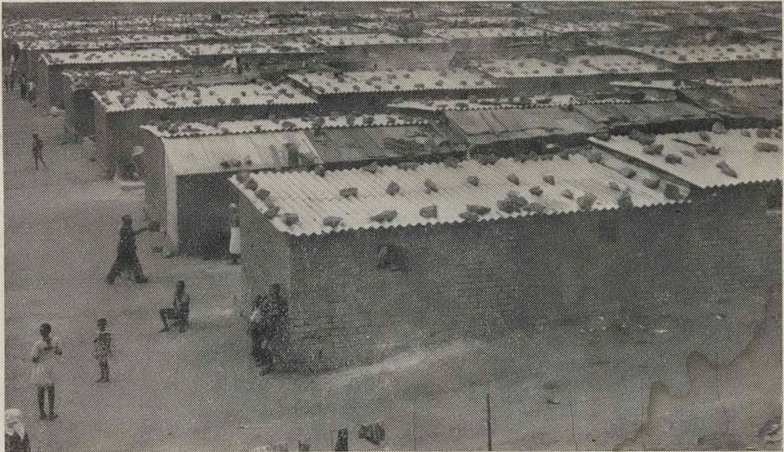
A general view of the Orlando Breeze Block "temporary" shelters.
