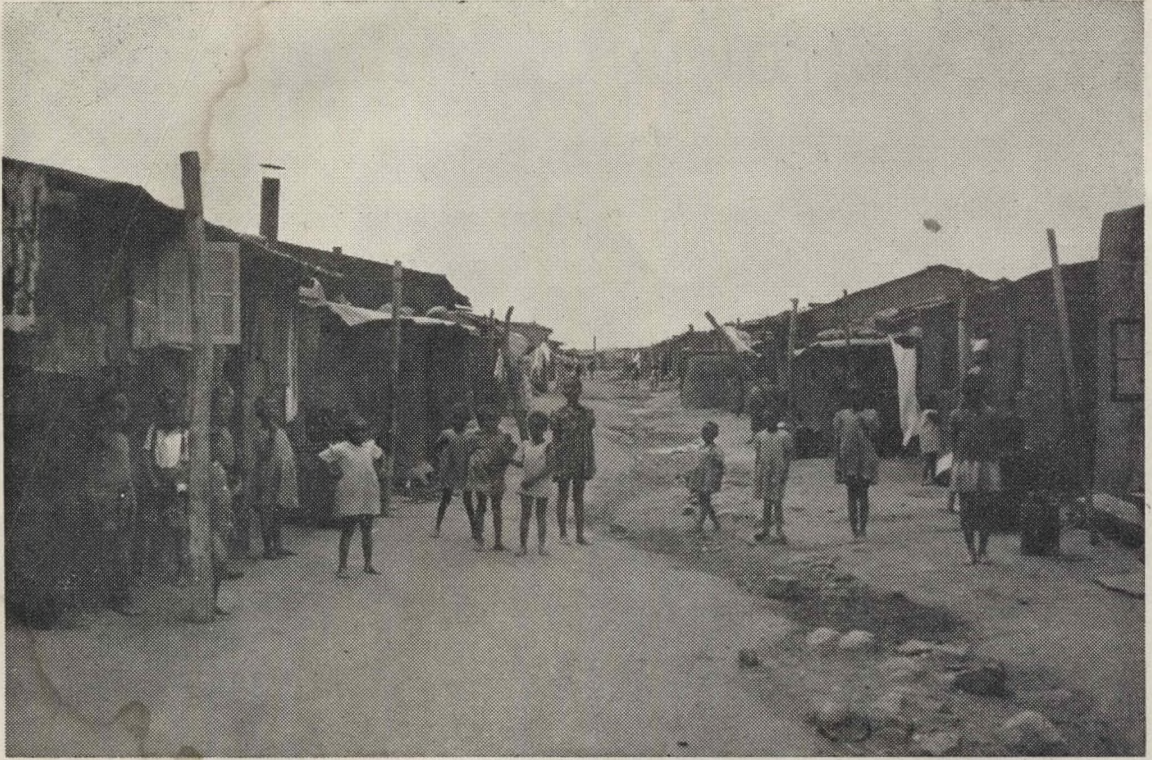
A street in Moroka with its all-purpose drain, in which domestic soilwater and stormwater flow together.
