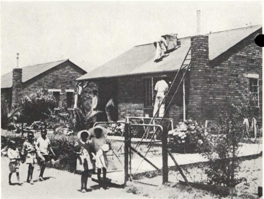
Maintenance of houses in Orlando West.
