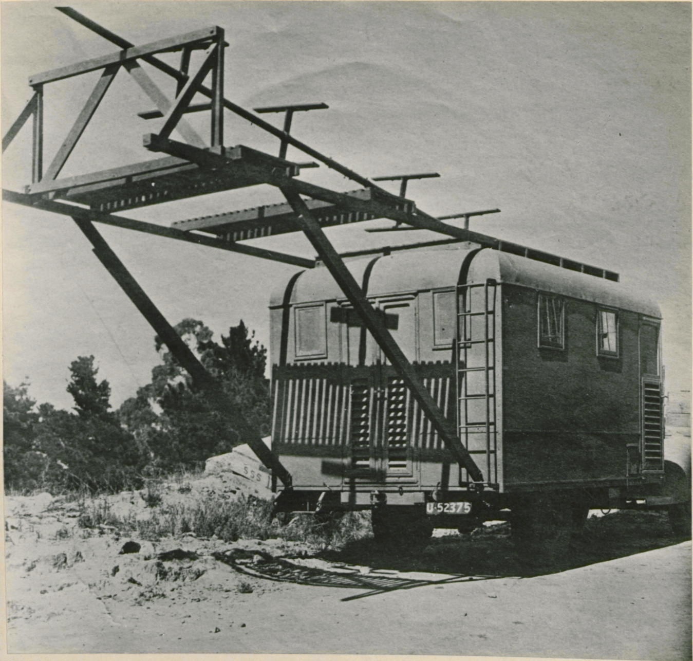
SPECIAL PLATFORM ON J.B.5 MOBILE FOR FACILITATING ERECTION OF THE AERIAL.
