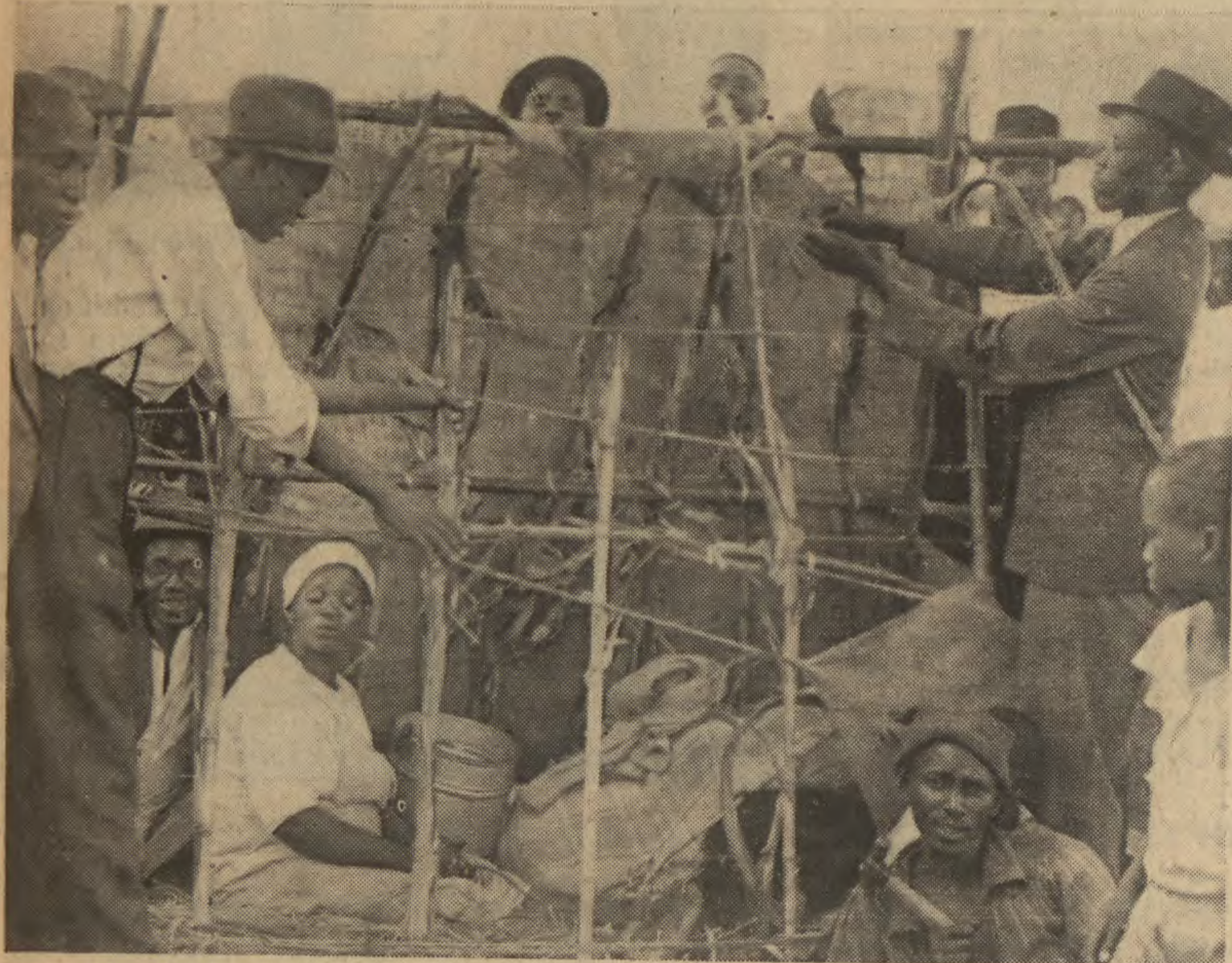
Men and women building a home in "Shanty Town" as a protest against the over-crowded conditions in Orlando Township. The Johannesburg City Council has agreed to erect "breeze block" houses as a temporary measure, in place of the shacks and huts built by residents.
